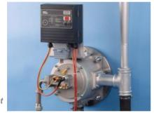
BCU on radiant tube burner
