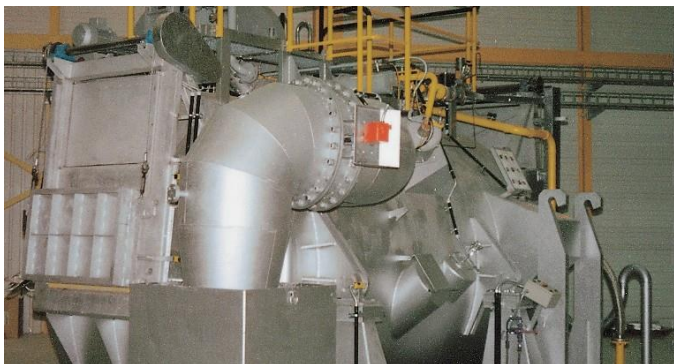
Aluminium tank furnace
