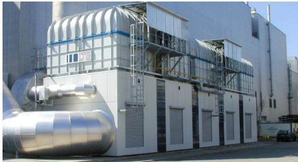
Incineration installation for thermal regenerative flue air purification
