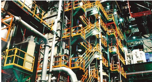
Strip galvanizing plant
