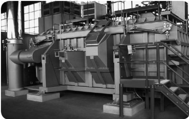
Aluminium industry: smelting furnace
