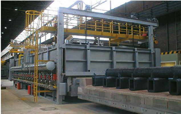
Metallurgical industry: bogie hearth furnace
