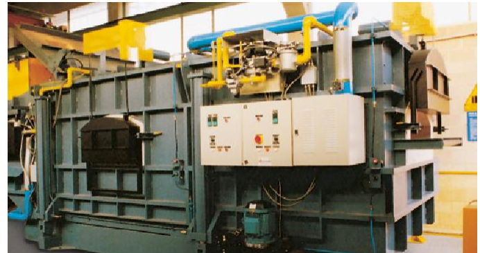
Air/gas ratio control on melting furnace for ensuring stoichiometric combustion over the entire capacity range
